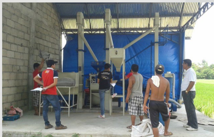
On-site installation and testing of Paddy Huller
